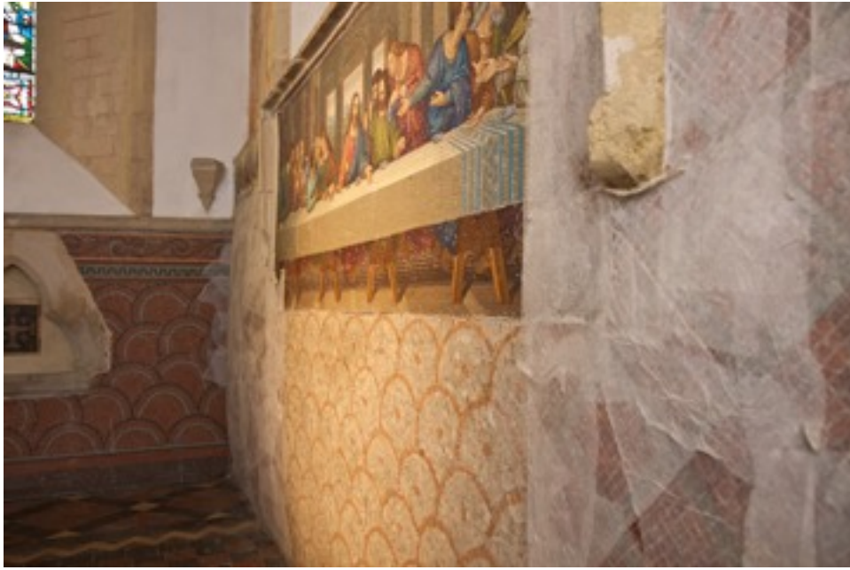
The etoline tissue applied in 1997 to support the mosaics
