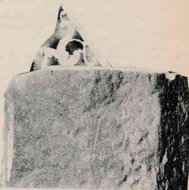
At Cheadle, Cheshire, parish church, the style is held in position by a supporting strap to prevent it from becoming detached from the dial.
