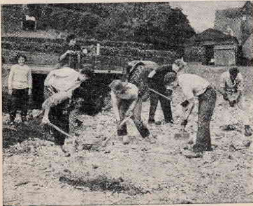
Constructing car park for Pembury Hospital, Kent
