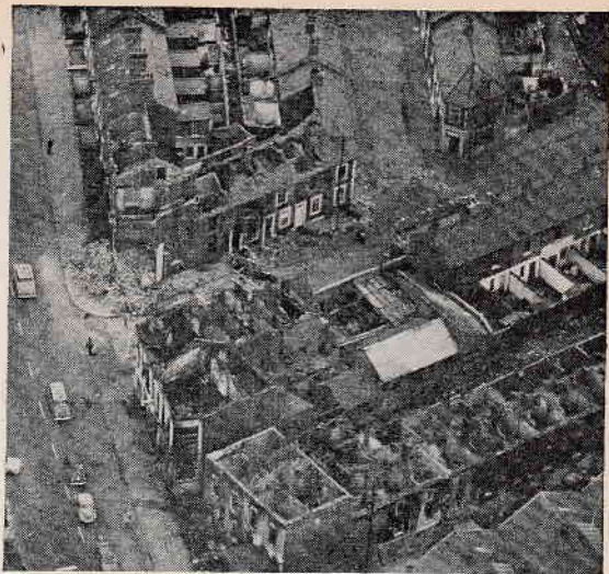
Falls Road area, Belfast after the strife — when hundreds of homes were destroyed.
